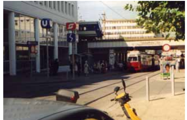
Interchange between the underground, the surface rail system, light rail, buses and taxis in Vienna, Austria
