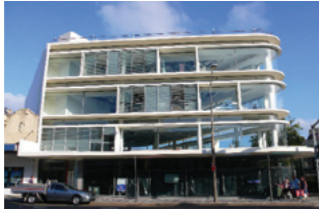
Sustainable office building, Double Bay Sydney
